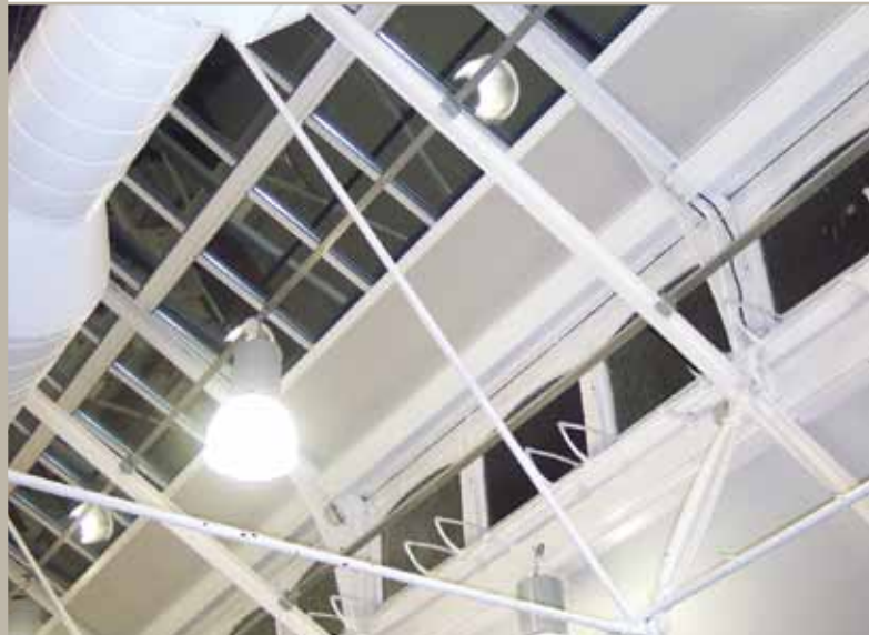
Fabric tension system (FTS) ensures fabric is held taut at all positions of the blinds
